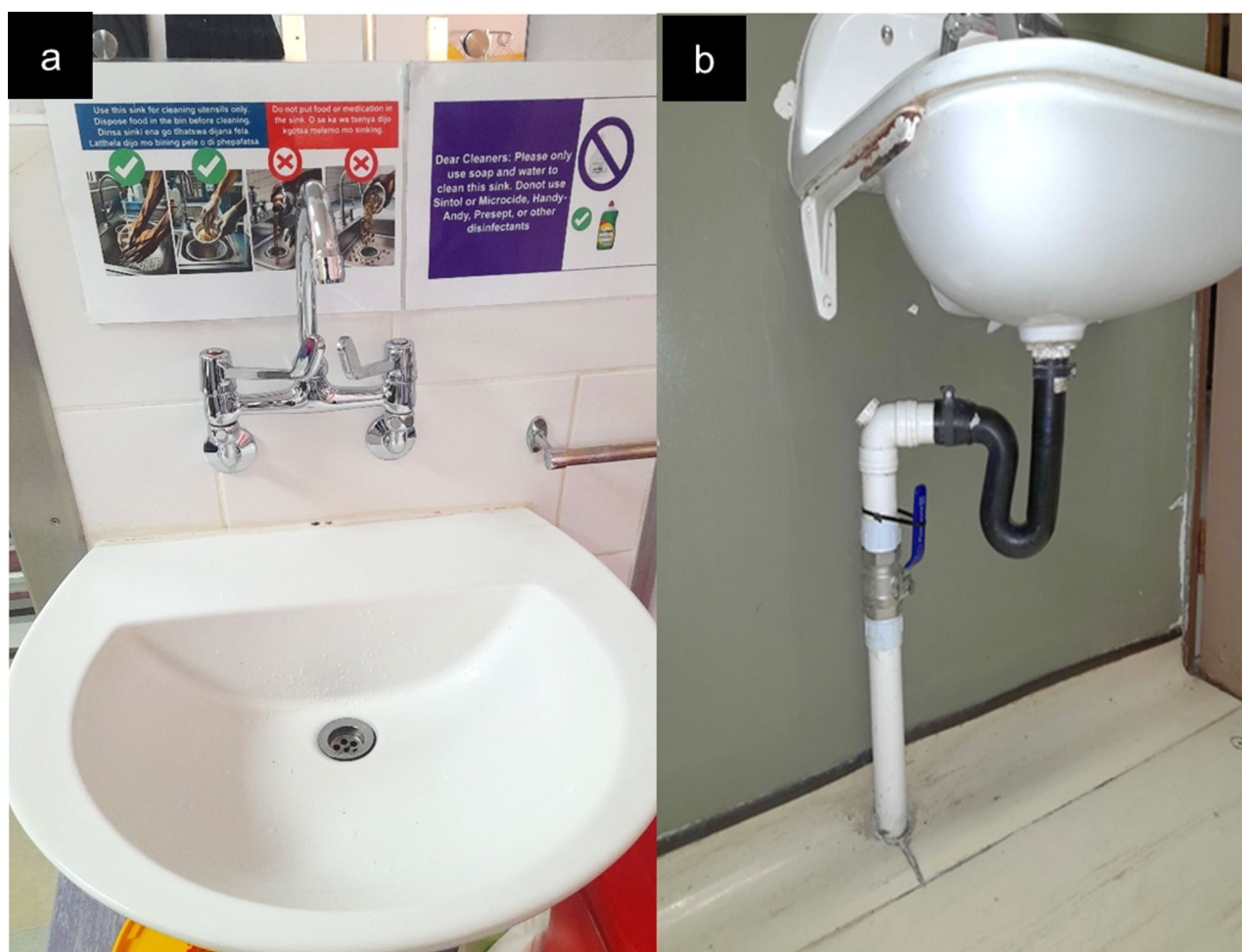
Fig. 2 Updates to hospital ward hand washing sinks to reduce drain contamination rates with drug-resistant Gram-negative organisms. Visual aids placed above sinks to indicate intended use (A) and installation of sink drain with ball valve on distal side of the trap to allow obstruction of flow and adequate contact time with disinfectant (B)
